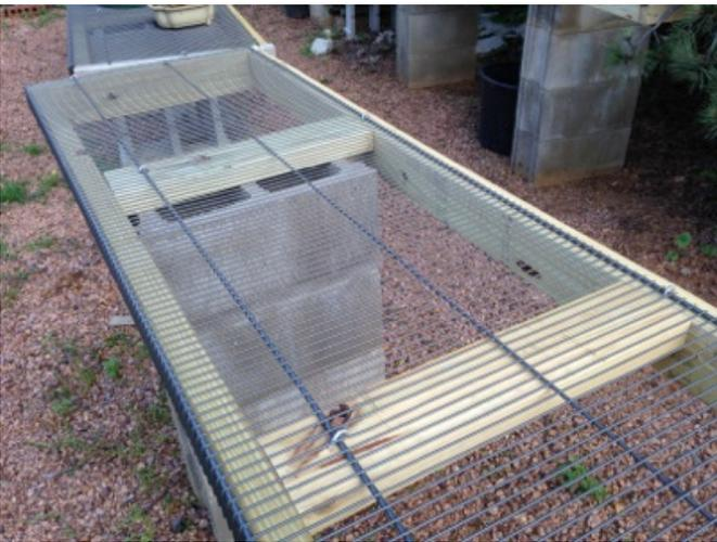
When all three braces are nailed on the one long side, place the other long side down and nail that in place.
